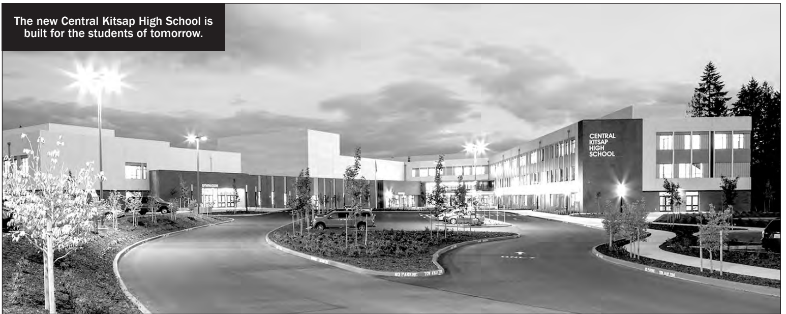
IMAGES COURTESY OF SKANSKA USA BUILDING
