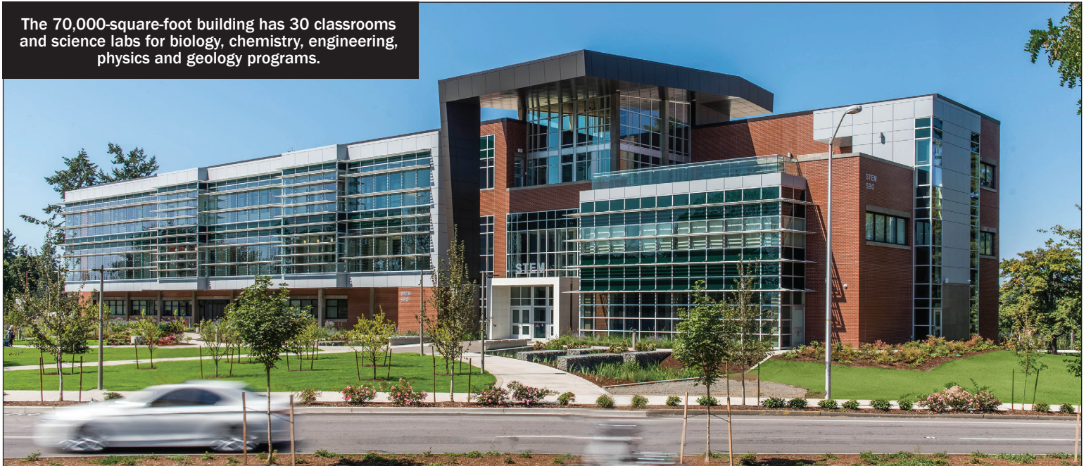
PHOTO BY MAX MIKHAYLENKO/VARIABLE VISUALS, COURTESY OF LSW ARCHITECTS
