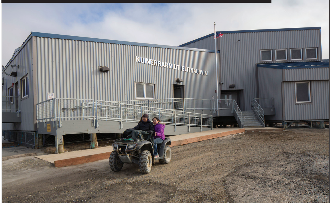
The K-12 school in Quinhagak underwent a renovation and 30,000-square-foot addition.
