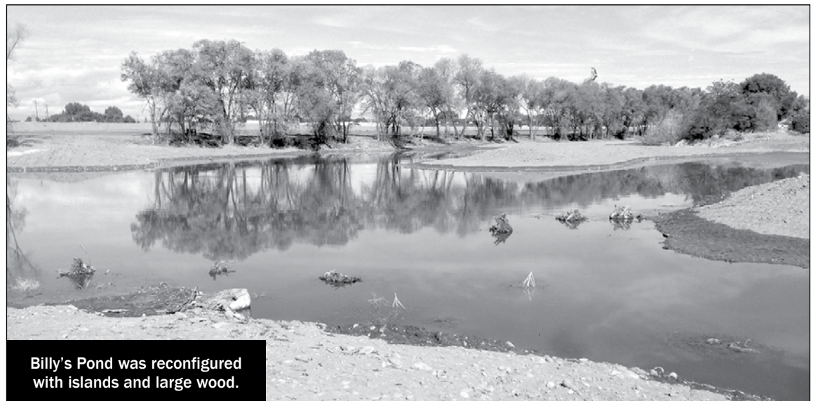
Crews excavated groundwater-fed channels near Billy's Pond.
