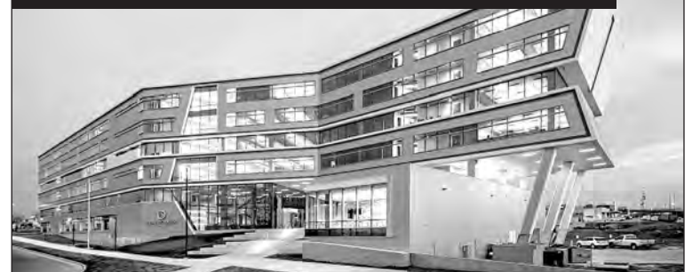
Lighting throughout Denver Water's campus was designed to support dark skies and limit light pollution with fully shielded fixtures that create a safe environment for after-hours use.
