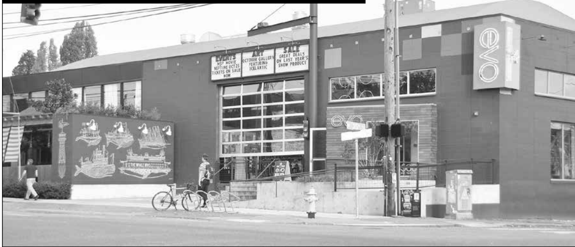
PHOTO FROM BAYLIS ARCHITECTS
