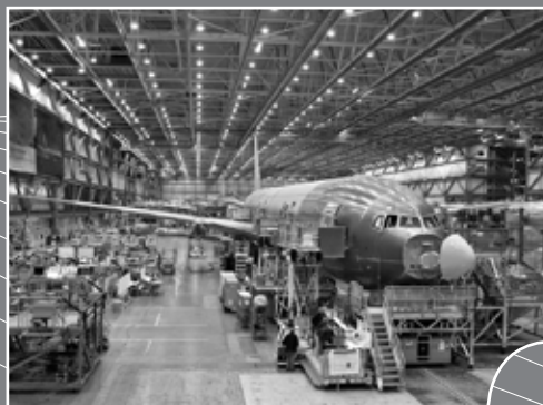
777 Moving Line Utilities, Building 40-025, The Boeing Company; Everett, WA
