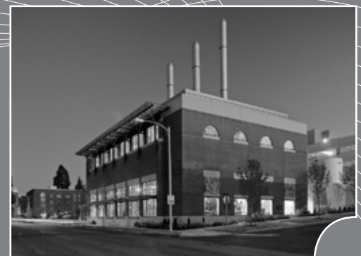
Central Energy Plant, MultiCare Medical Center; Tacoma, WA
