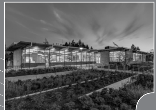
Support Services Center, LEED Gold Certified, Federal Way School District; Federal Way, WA
