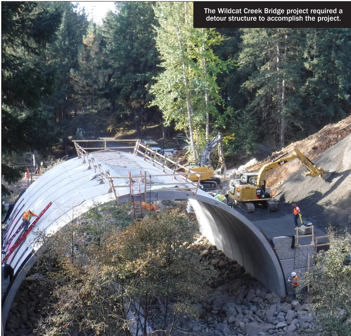
PHOTO PROVIDED BY GRAHAM CONTRACTING
