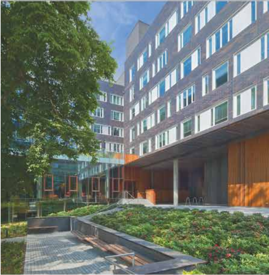
UW Elm Hall LEED Gold
