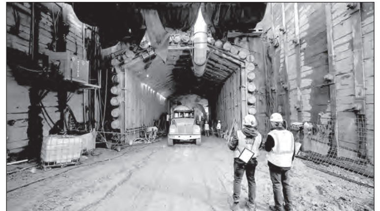
The new arena is served by a 25-foot-wide tunnel, which provides enough room for two passing semi-trucks.
