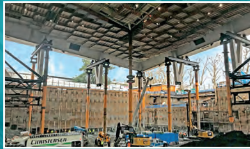
Raise the roof to allow a 600,000-cubic-yard excavation
