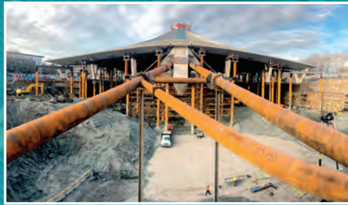
Design temporary supports for a 44-million-pound seismically upgraded historic roof
