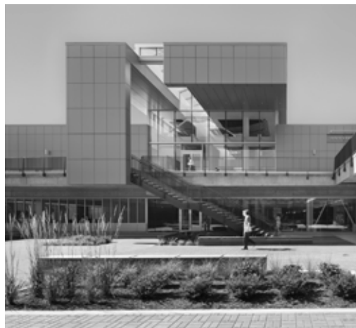
Health Sciences and Student Resources (HSSR) Building North Seattle College, Seattle, WA
