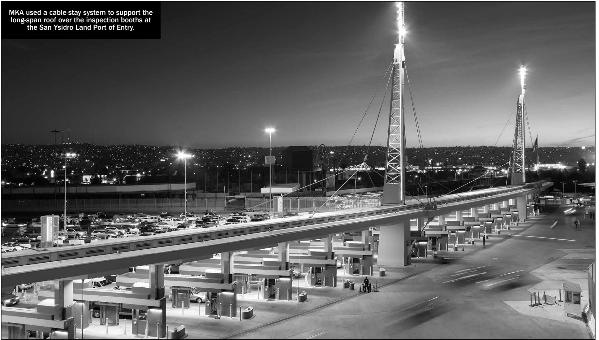
PHOTO COURTESY OF MAGNUSSON KLEMENCIC ASSOCIATES
